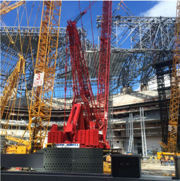
Large Cranes 600 Ton Lifts
